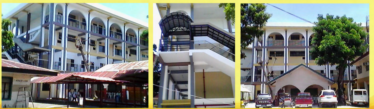
Completion of the 3-Storey Business Center Building with Mezzanine located at the TSU Main Campus.
